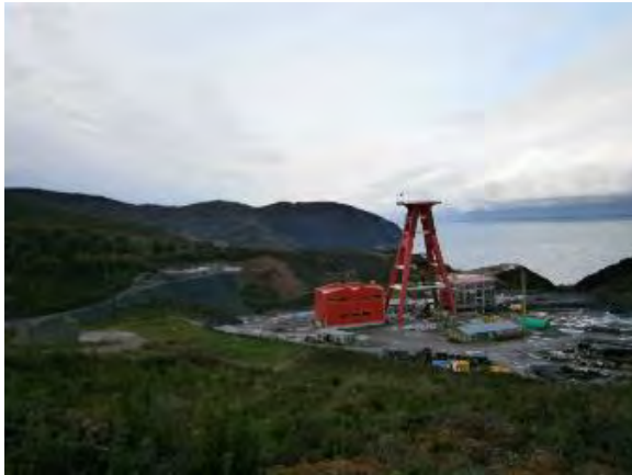
Photo 2. General view of the Shaft-1 site
