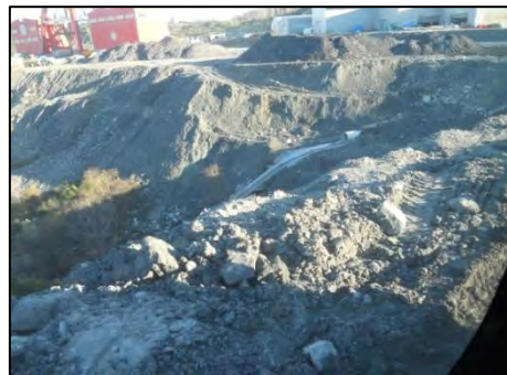
Photo 5.4. Capak Creek reclamation
