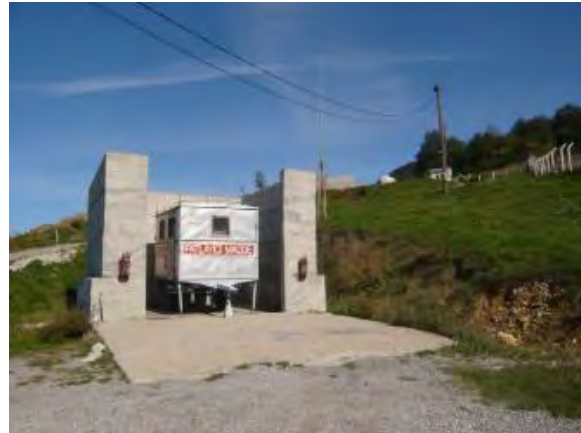
Photo 3. Magazine (explosive warehouse)
