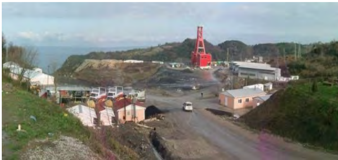
Photo 1. Main Project Site and Shaft-1 View
