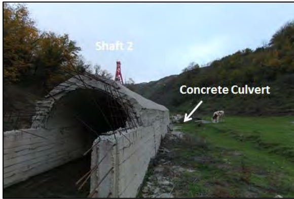
Photo 5.6. Reinforced Concrete Culverts for Buyukdere Creek
