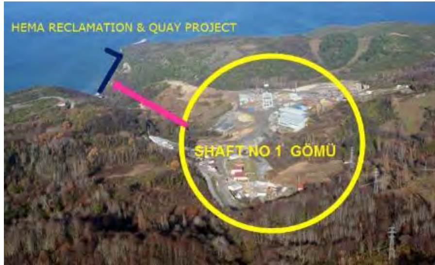
Figure 2-27: Location of the port with respect to the Shaft-1 area
