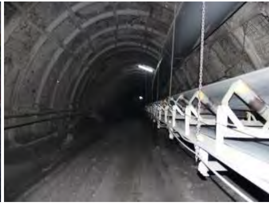
Photo 7. Surface inclined gallery
