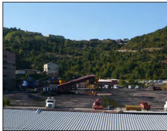
Photo 5.10. View of TTK Shaft Area
