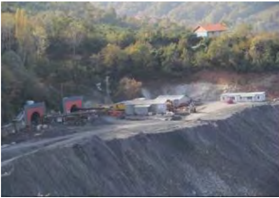
Photo 6. Surface inclined gallery entrance
