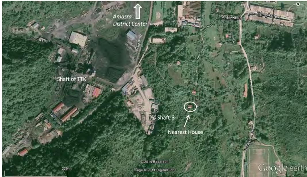
Figure 5-5: Overall view of Project components around Shaft-3 area
