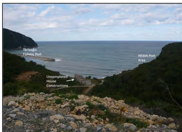
Photo 5.11. The Uncompleted House Constructions and HEMA Port Area
