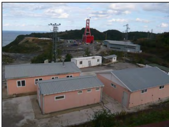
Photo 5.5. General view of Shaft-1 area
