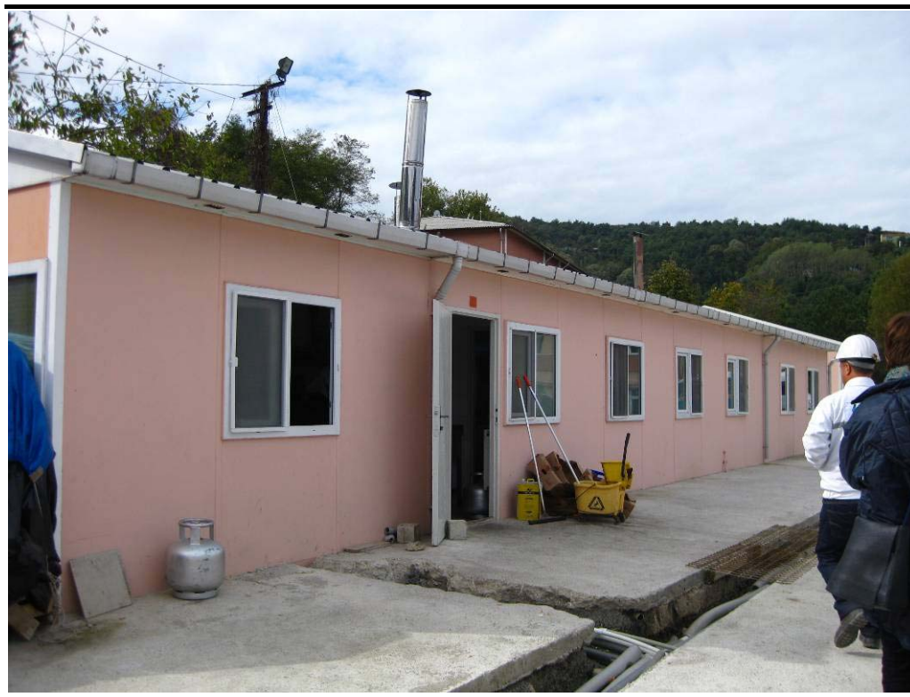
Photo 28 Central kitchen operated by Hema at Shaft # 3.
