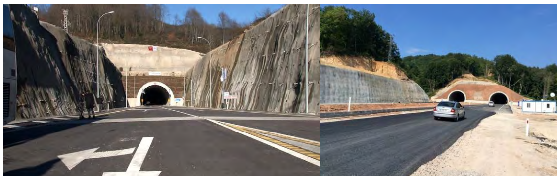
Figure 12-7: Amasra-Topderesi road and tunnel
